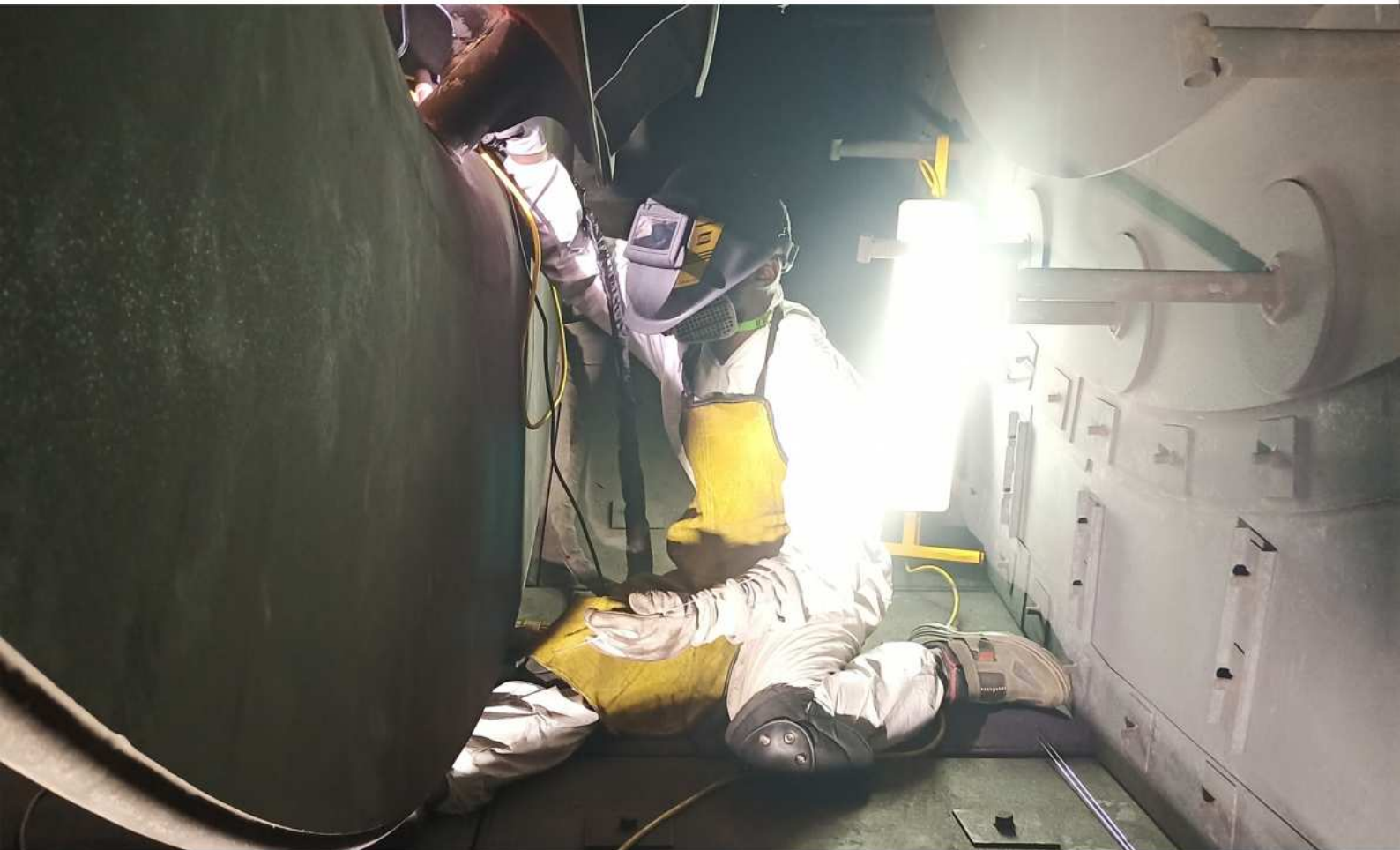
EXHAUST DIFFUSER CRACK REPAIR WORKS
