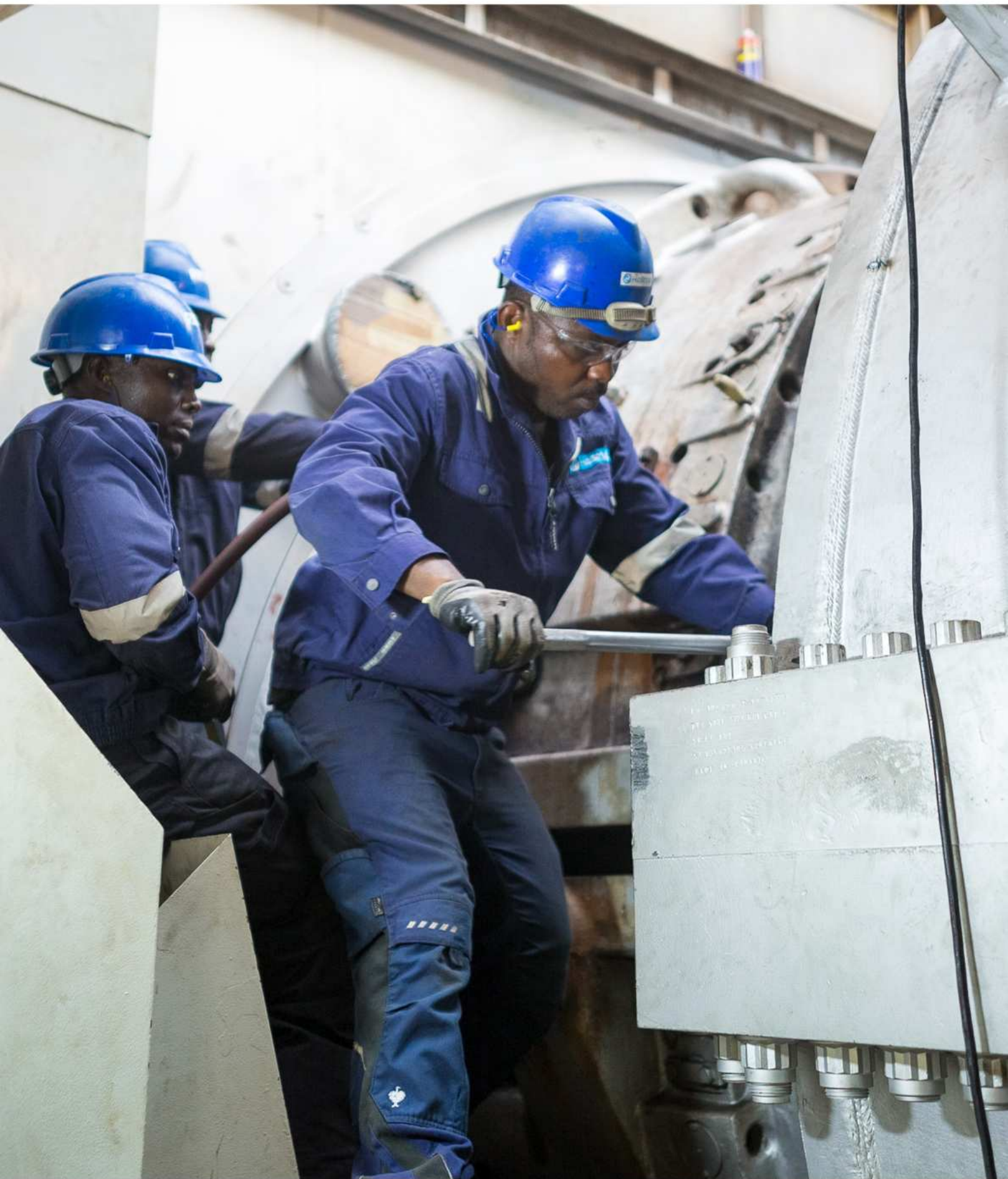
GAS TURBINE CASING
